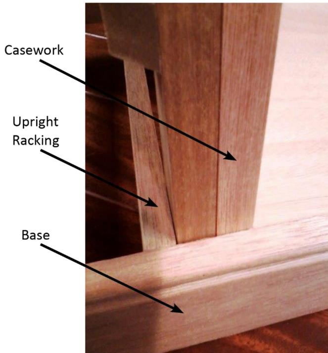
Figure 66: Faceframe with Racking
