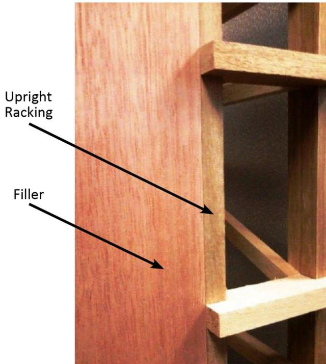
Figure 64: Filler for Racking at the Base
