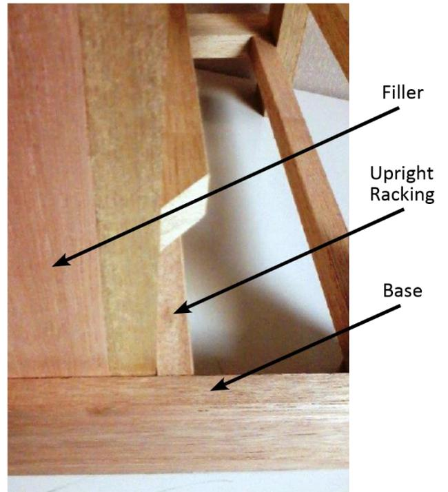
Figure 65: Casework with Racking
