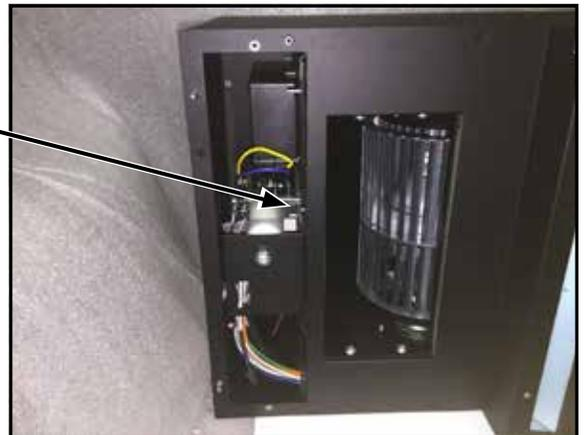
**25** Re-install the electrical panel using the 2 Phillips head screws removed in step #7.
