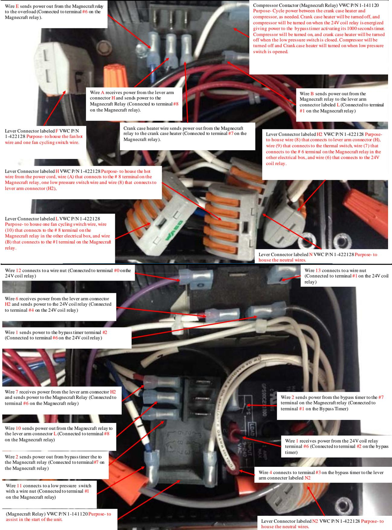
Wire E sends power out from the Magnecraft relay to the overload (Connected to terminal #6 on the Magnecraft relay).
