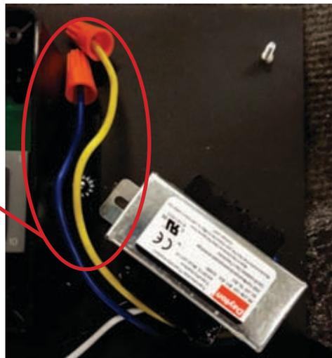
**Condensing Unit:** Connect the other end of the 18-2 low-voltage thermostat wire to the grey and purple wires located in the grey electrical box on the condenser skid.
