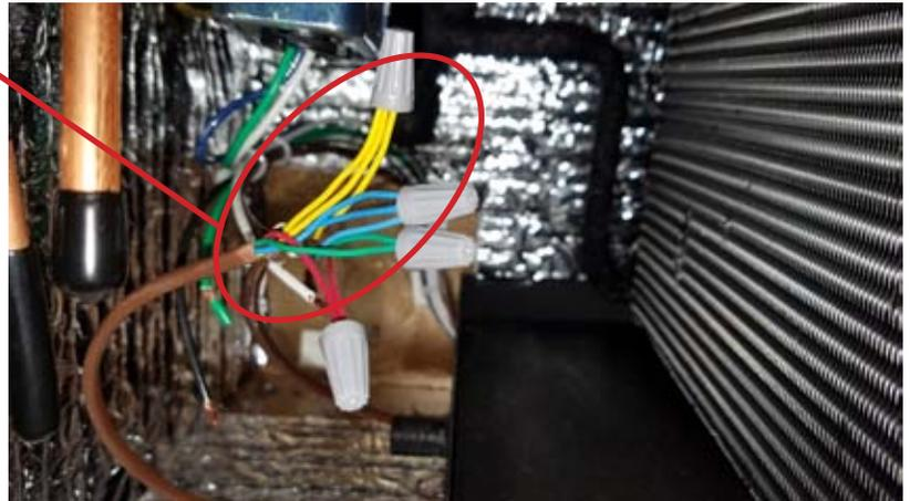
**Condensing Unit:** Connect the other end of the 18-2 low-voltage thermostat wire to the grey and purple wires located in the grey electrical box on the condenser skid.
